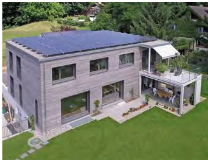
Figure 30. Picture of PV plant on a building. Source:
